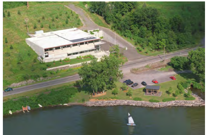
Cornell University's Lake Cooling System. Credit: Jon Reis Photography, used with permission of Cornell University.
